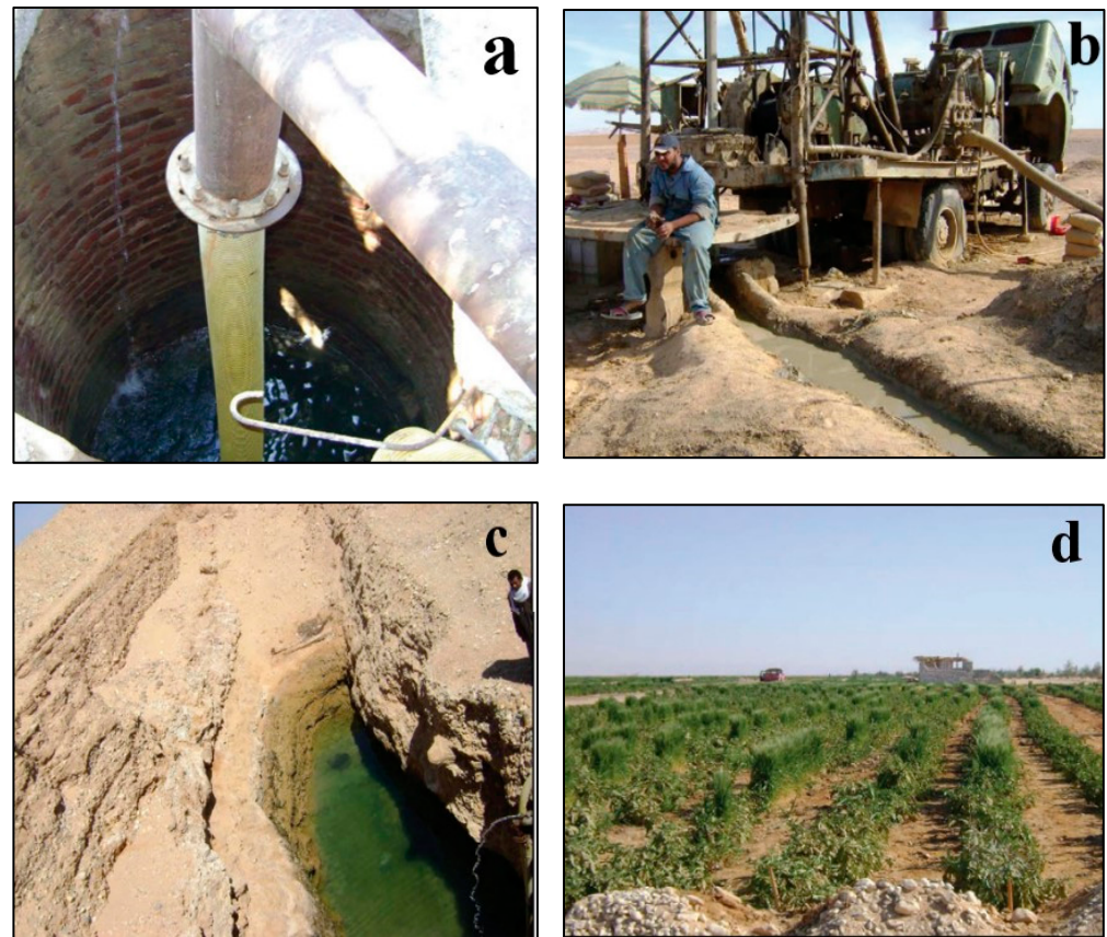
Figure 7. Field photographs of the study area: (a) a highly productive well with 4 m depth; (b) well drilling at central Wadi Qena Basin to a depth of 120 m; (c) excavated water well at inter-bedded sand and gravel, bounded by shale; (d) corn and tomato crops at the southern part of Wadi Qena Basin.
