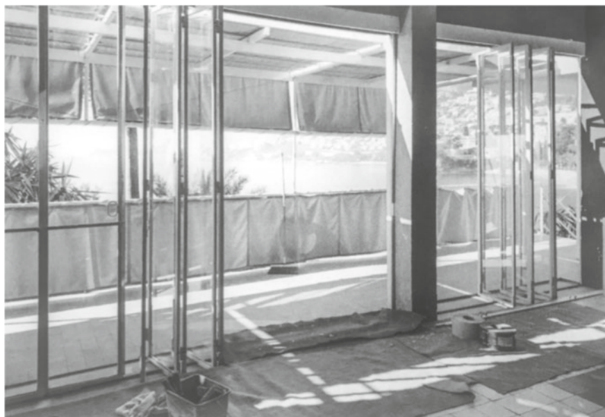
Fig. 2 Detail of ribbon windows with a screen-like opening system, Villa E.1027, Roquebrune-Cap-Martin. Picture by Kasper Akhøj (Akhøj, 2017)
