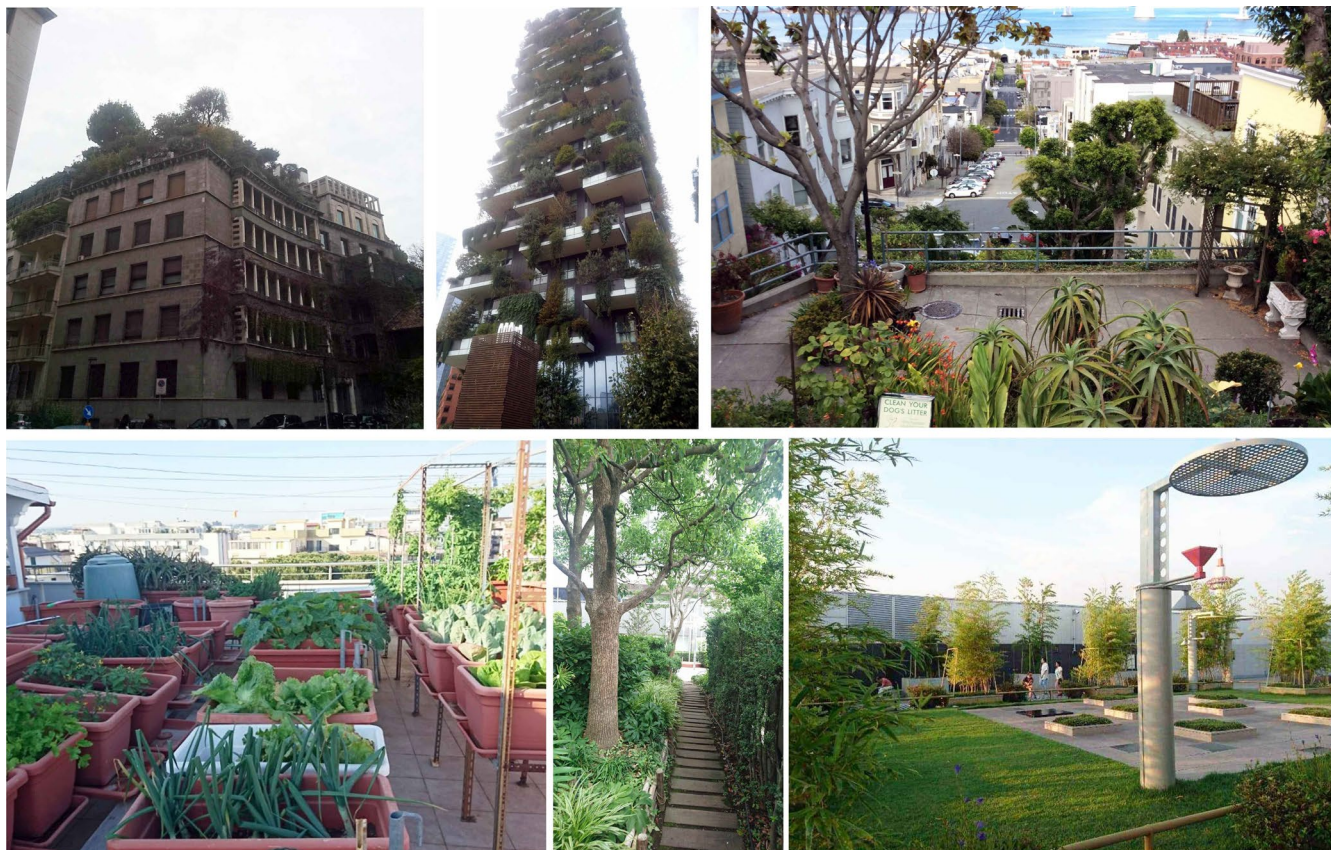
FIGURE 9 Urban green roofs. (Top row) from left to right: green roofs in old buildings (Milan, Italy); vertical forest skyscraper (Milan, Italy); garden terraces (San Francisco, USA). (Central row) from left to right: 'food roof' with vegetables (Trani, Italy); Mohri Garden at Roppongi Hills (Tokio, Japan); green roof of Kyoto railway station (Japan). Pictures by Adriano Sofo
