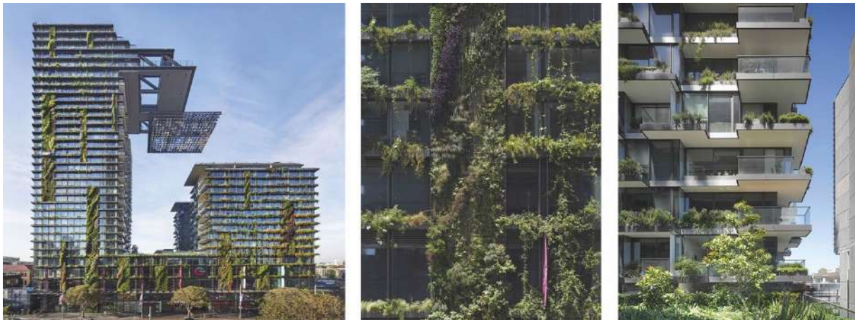
Fig. 5: One Central Park, Ateliers Jean Nouvel, Sydney, Australia (© Ateliers Jean Nouvel, www.jeannouvel.com )
