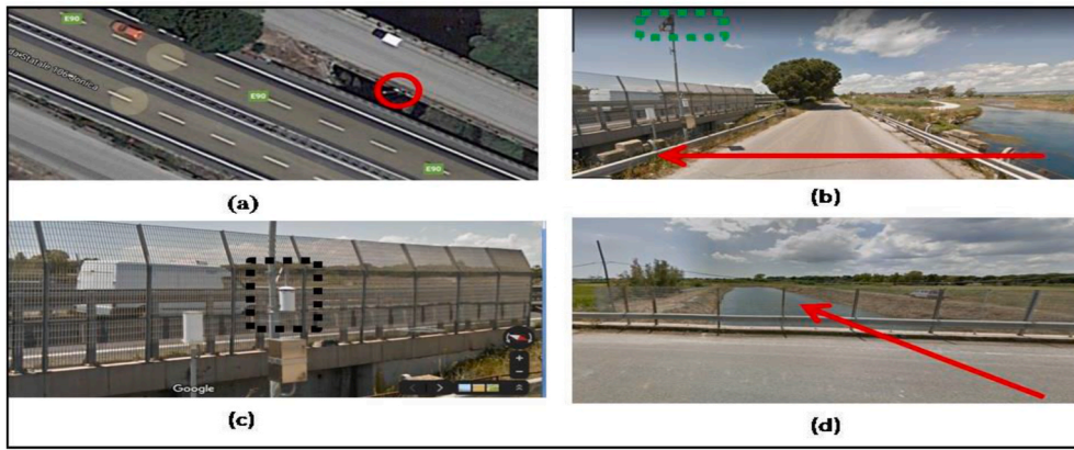
Fig. 5. Sensing system for river level detection: (a) location on the bridge, (b) flow direction, camera and PV power panel, (c) ultrasound level sensor, (d) water flow direction downstream of the bridge.
