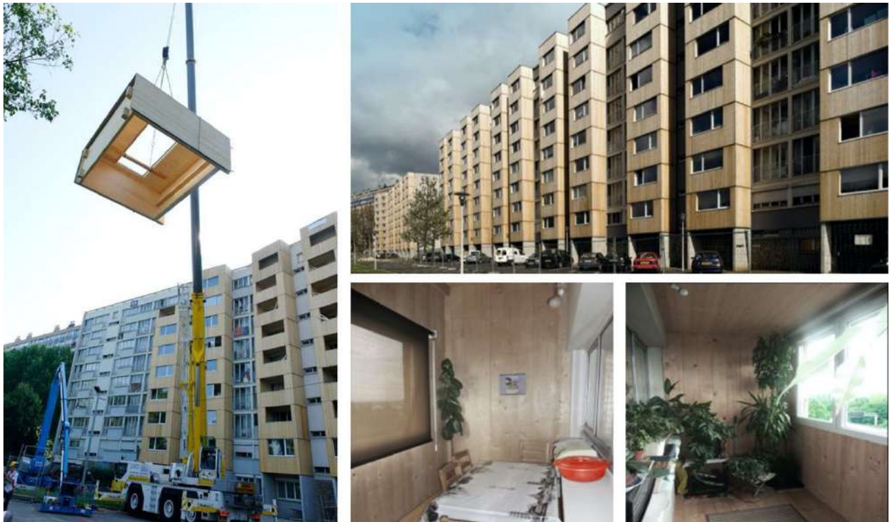
Fig. 3: Retrofitting practice of Loggias Bondy, Paris (credit: Studio Virtuel Architecture, http://www.virtuel.fr/ )
