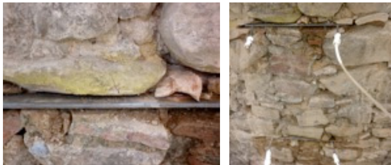
Figure 6: Double flat-jack test and masonry characterization.
