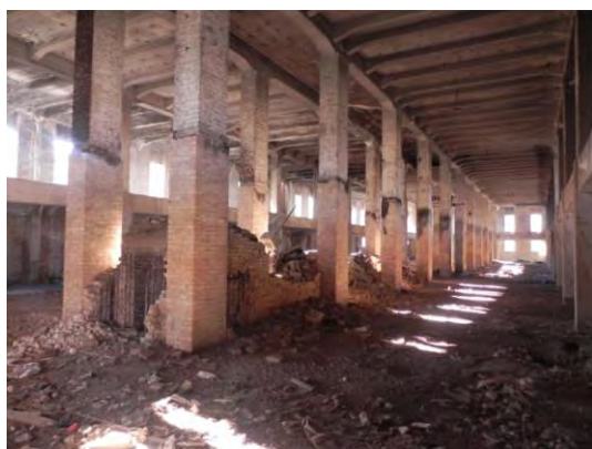
Plate 2 – The central nave
