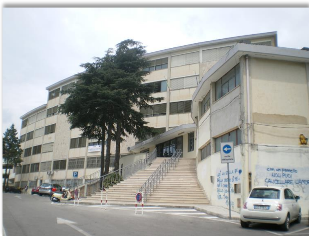
Figure 3. Building envelope of Liceo Classico E. Duni
