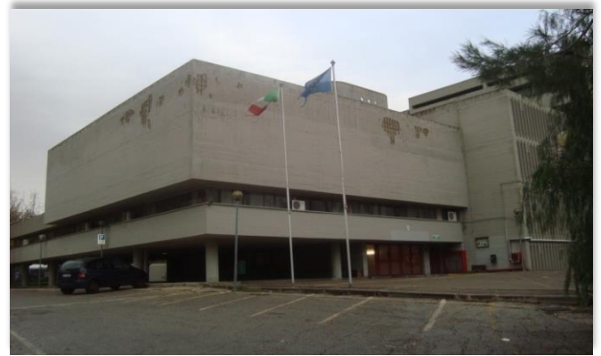
Figure 4. Building envelope of Liceo Scientifico D. Alighieri
