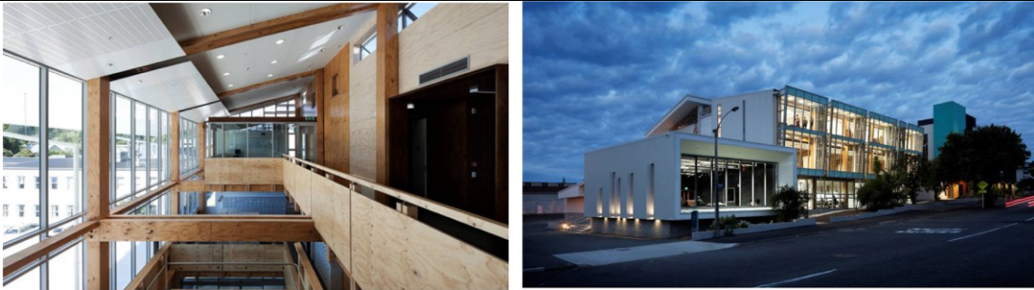
(a) Internal and external view of NMIT Arts and Media Building, Nelson, NZ [77].
