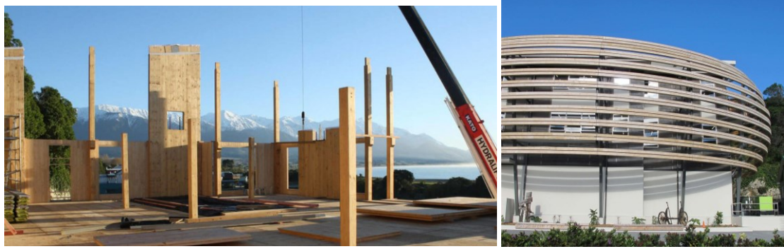
(h) Construction and external view of Kaikoura Civic Centre in New Zealand [81]
