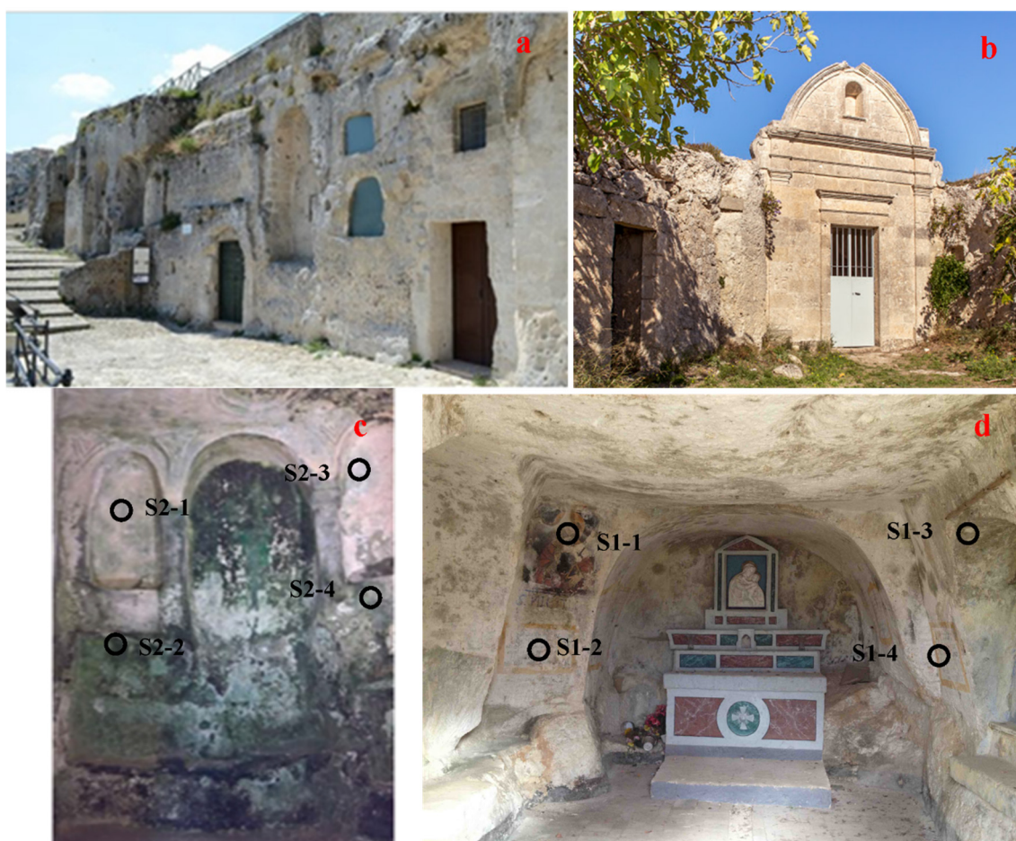
Figure 1. General view of the environmental context (a,b) and interior (c,d) of the two rupestrian churches “Santa Lucia alle Malve” and “La Madonna dei derelitti”. Photos from the interior (c,d) of the two rupestrian churches also show the S1-1, S1-2, S1-3, S1-4, S2-1, S2-2, S2-3 and S2-4 sites from where non-invasive sampling was performed. To investigate overall fungal species present, material from four sampling points of each site was combined into two samples corresponding to (A) “Santa Lucia alle Malve” church and (B) “La Madonna dei derelitti” church.
