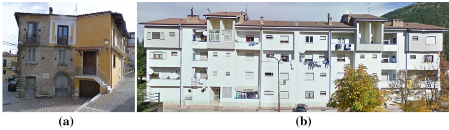
Fig. 2 a Example of ensemble of masonry buildings; b example of ensemble of RC buildings in the study area in their typical arrangement
