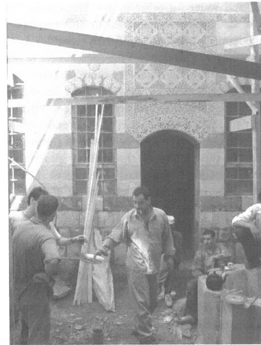
Figure 7. Tea break at the Bayt Montlucon restoration site.
