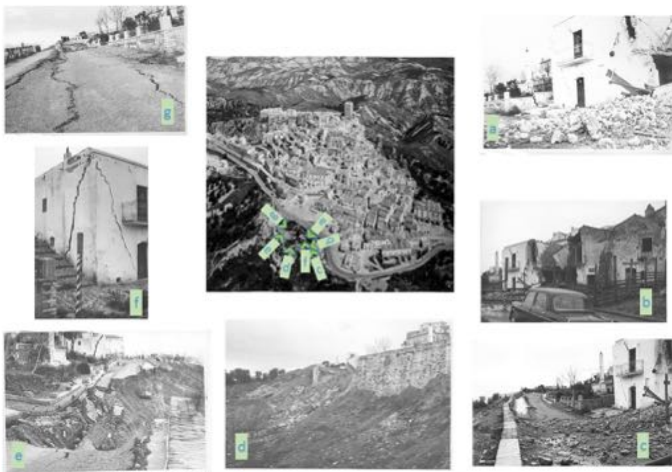
Fig. 14 Photos of damage caused by the 17 January 1965 landslide event. The green boxes show the view angle of the historical photos taken in the aftermath of the parossistic event. Image in (e) shows the landslide niche upstream the retaining wall so testifying the retrogressive features of the
