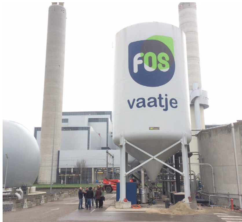
Figure 2. Phosphorus recovery from sludge at pilot plant of the Amsterdam water board Waternet Source: JE Jansma.
