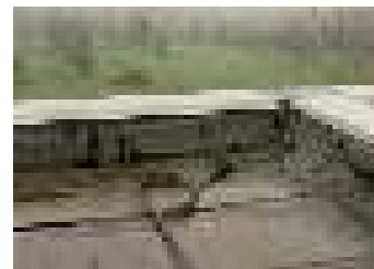
Figure 112 – Perpendicular ridgings caused by reptation. The two layer of the membrane are crossway installed
