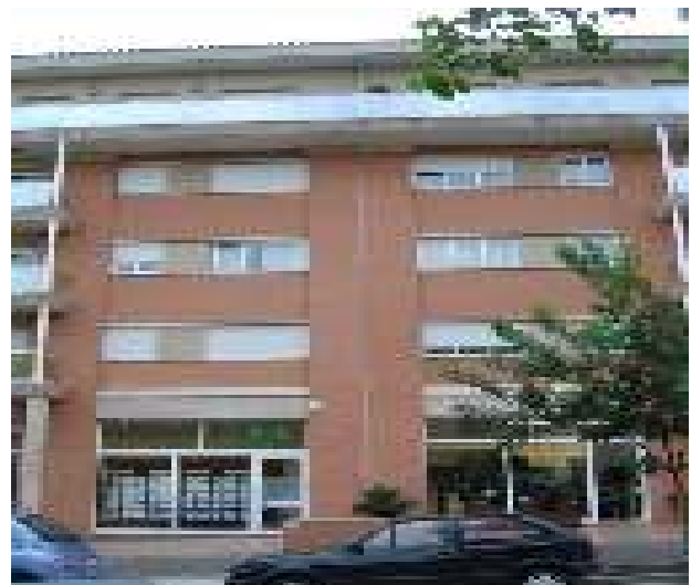
Figure 15 – View photo of a set of newly constructed residential buildings in urban peripheries
