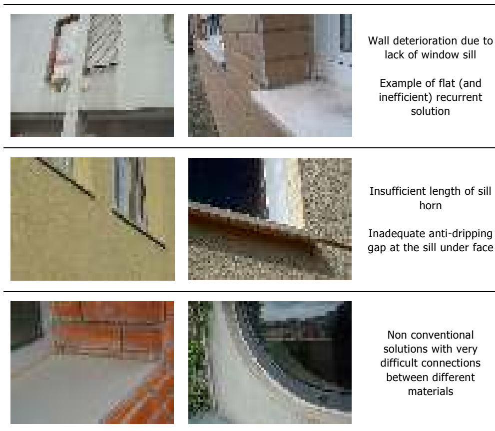
Figure 67 – Examples of window sills with different shapes and materials, which functional performance is somehow compromise
