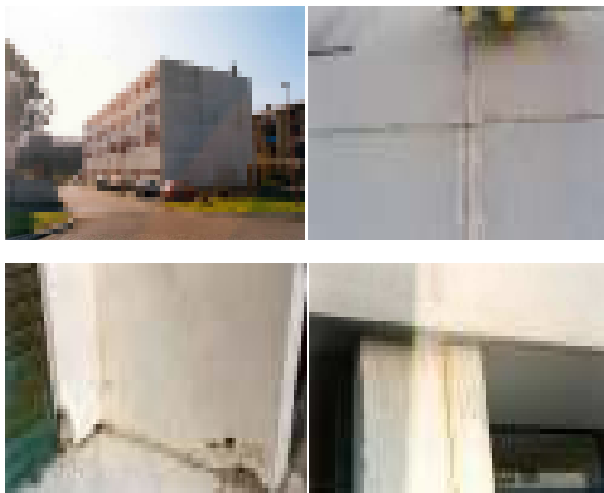
Figure 161 - Pozzuoli (Napoli), Monterusciello n. 148 flats of subsidized buildings realized with large bearing panels
