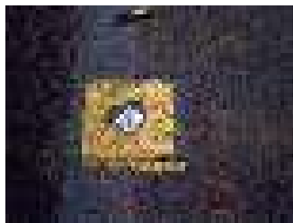
Figure 113 – Puncturing by mechanical fasteners
