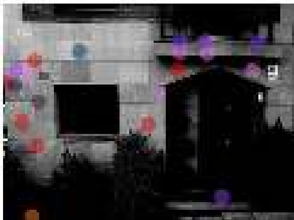
Figure 23 – Planimetry based on photographs to facilitate identification, census and classification of anomalies detected in the natural stone façade placated by a group of single houses
