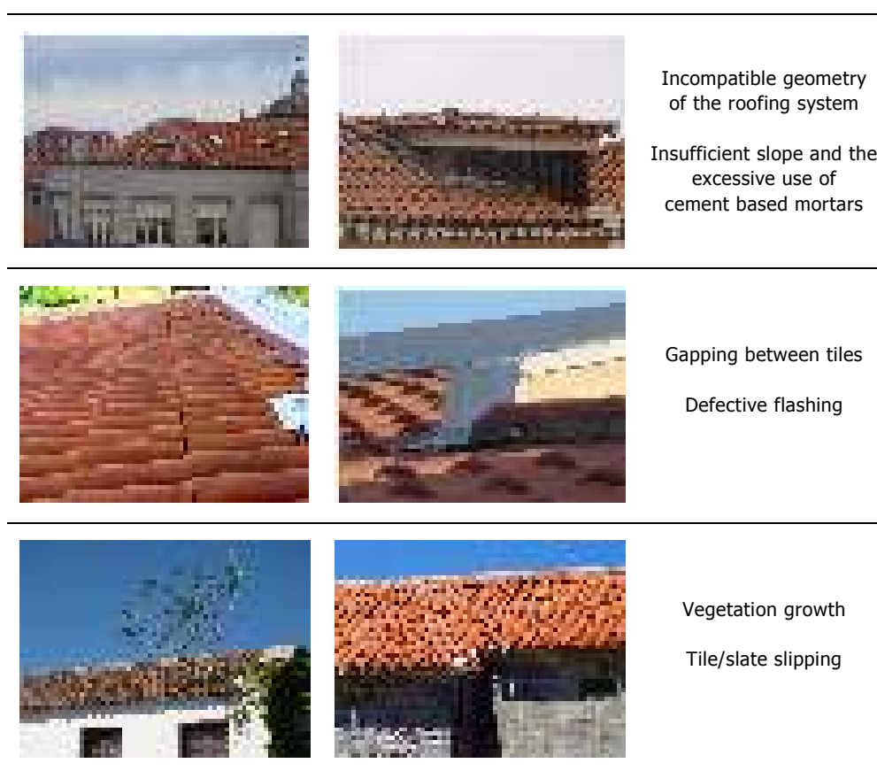
Figure 68 – Examples of defects for pitched roofs
