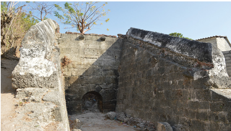
Figure 6: The kiln for baking the block.
