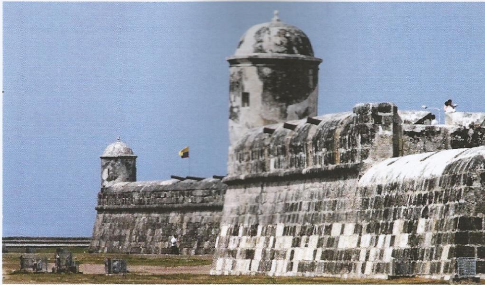
Figure 9: The sighting tower of the wall.
