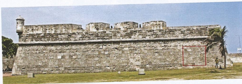
Figure 4: 'Santa Catalina' bastion.
