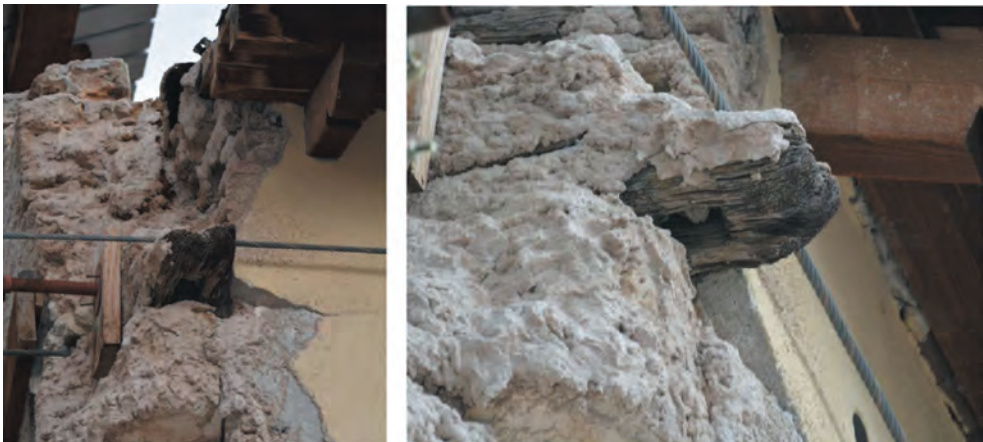
Figure 1: Wooden chains placed inside the wall. Building in Piazza San Domenico.
