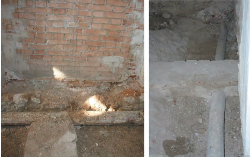
Figure 2: Wooden chains placed outside the wall of Palazzo Zuzi.
