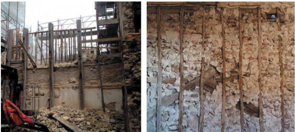
Figure 7: The 'hut' technique in individual wall panels of buildings in Via delle Aquile.
