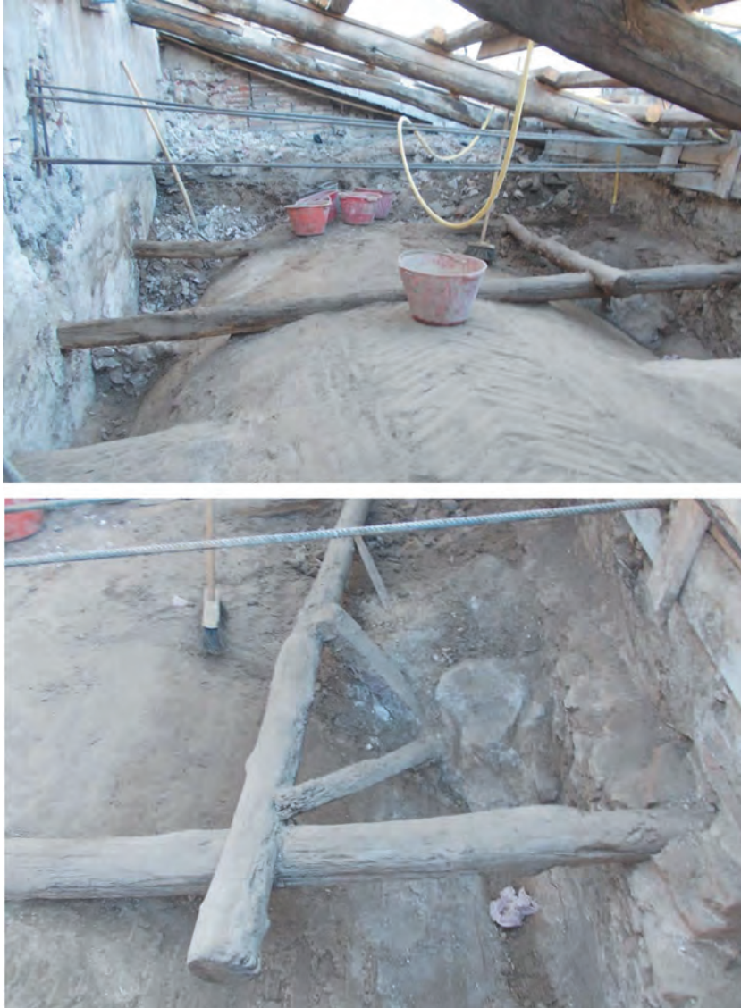
Figure 3: Palazzo Gualtieri. The transverse chains are longitudinally contrasted by rafters where retaining elements, embedded in the abutment, are connected.
