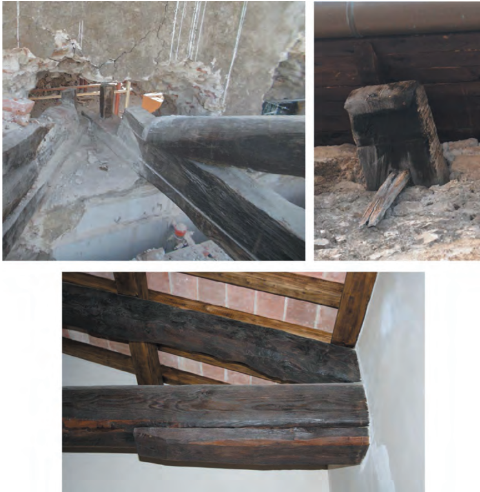
Figure 5: Details of the support knot solution in Palazzo Farinosi.
