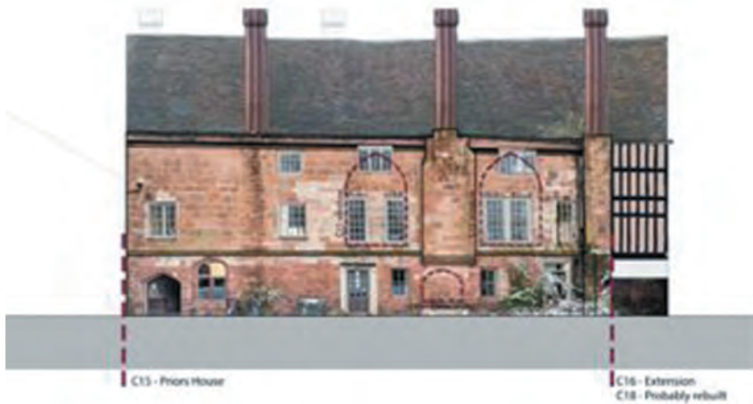
Figure 8: Photo elevation and analysis of East elevation.
