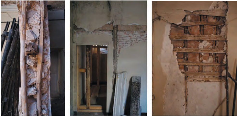
Figure 8: Light partitions attributable to the 'hut' technique in Palazzo Ardinghelli.
