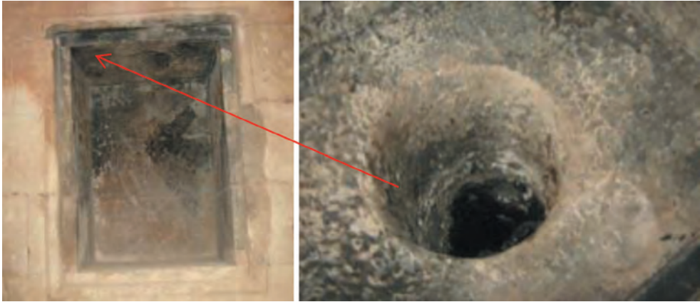
Figure 2: A niche (left) and its ventilation hole (right) on one of the walls in İshak Paşa Palace, used for candles (photo: author's archives, 2011).
