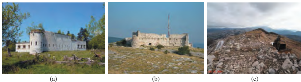
Figure 7: Different examples regarding the state of preservation: ‘good’ – ‘damaged’ – ‘destroyed’. (a) Fort IV Pasin brdo, Sarajevo (2011). (b) Fort 6, Mostar (2015). (c) Guardhouse Goli Vrh, Krivošije (2008).
