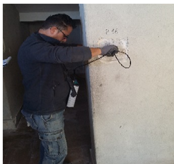
Figure 2. Ultrasonic test performed to column 16.
