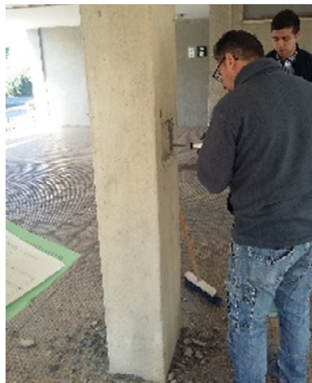
Figure 1. Sclerometer test performed to column 24.
