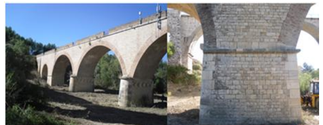
Figure 5. Some photos of the Cavone Bridge.
