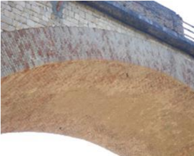
Figure 2. Particular of a main brick masonry arch.
