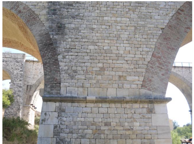
Figure 4. Spandrel wall of regular stone blocks.
