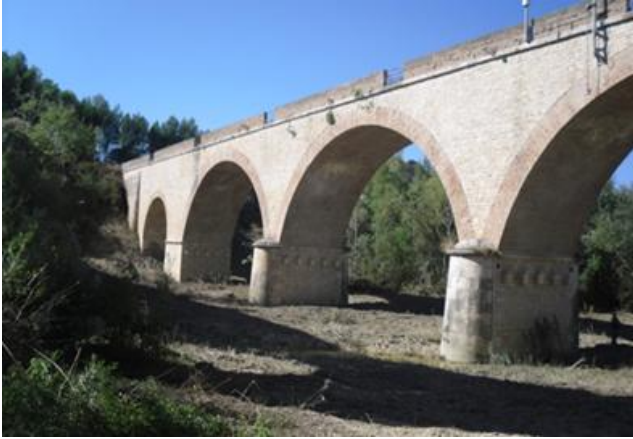
Figure 1. An overview of Cavone Bridge.
