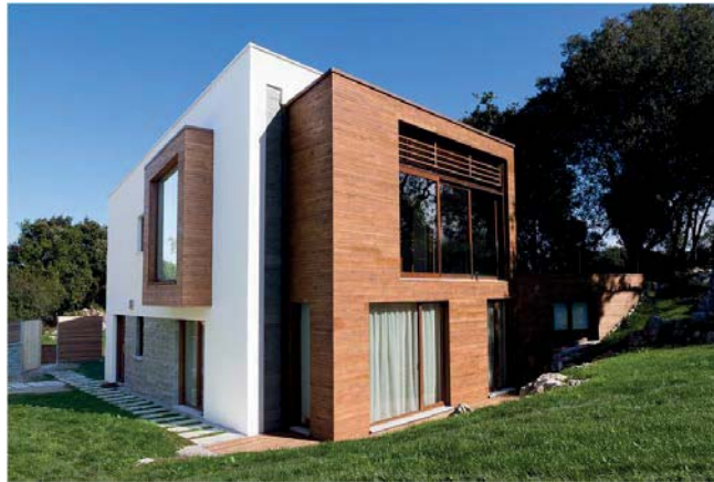
Figure 1: View of thermally modified Radiata Pine wood elements in a passive house.
