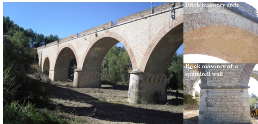
Figure 6 – Some photos of Cavone Bridge
