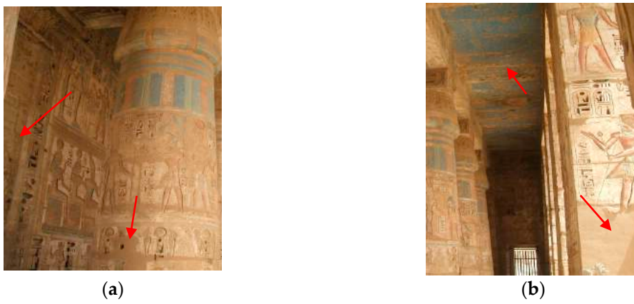
Figure 8. The walls Deterioration in Medinet Habu temple (a,b).
