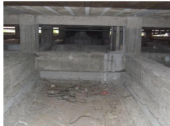
Figure 4 – Foundation of classrooms buildings
