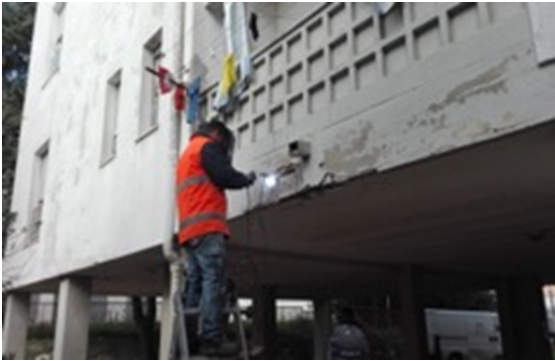
Figure 6. Extraction of steel to the beam 23-29.
