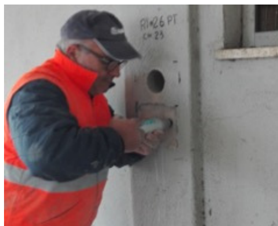
Figure 4. Sclerometric test performed to column 26.
