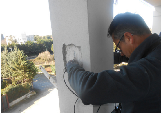
Figure 5. Ultrasonic test performed to the column 21.
