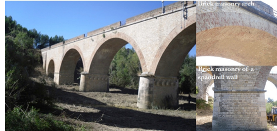
Figure 7. Some photos of the Cavone Bridge.
