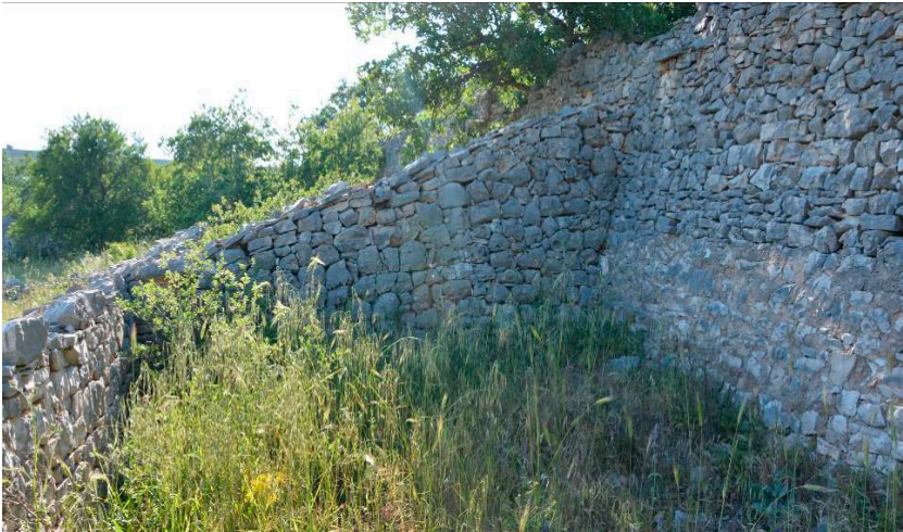
Figure 12. Jazzo “Del Demonio” —Dry-stone constructions.
