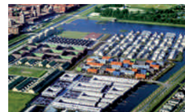
MVRDV, Hagen Island Housing, Ypenburg, 2000-03
