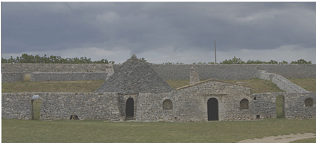
Figure 1. Dry-stone rural buildings with stone walls for the delimitation of borders between neighboring countryside estates.
