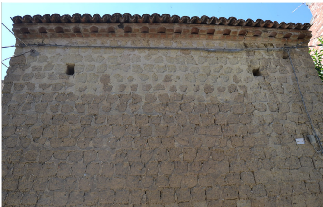
Figure 2. Earthen rural construction realized with adobe bricks.
