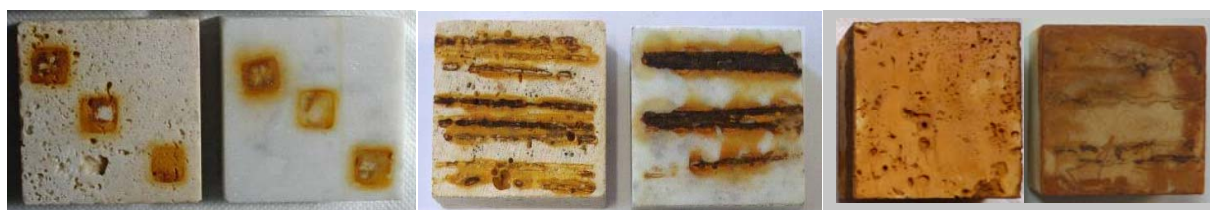
Figure 1. Evidence of corrosion induced Iron stains on Carrara and Travertine reference stones.
