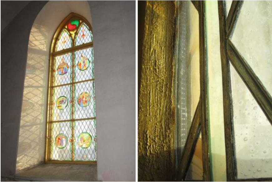
Fig. 21 A modern glazing unit on the exterior side of the historic window preserves the original appearance while reducing thermal conductivity and air leakages
