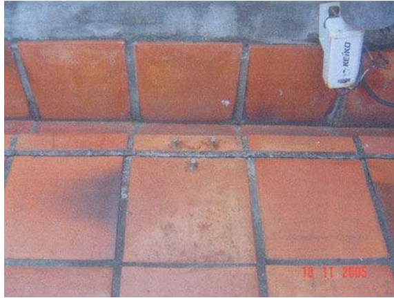
Fig. 17 Monitoring station and pins fixed to the south terrace, fifth floor (Nov 2005 —Cerme Engenharia)
