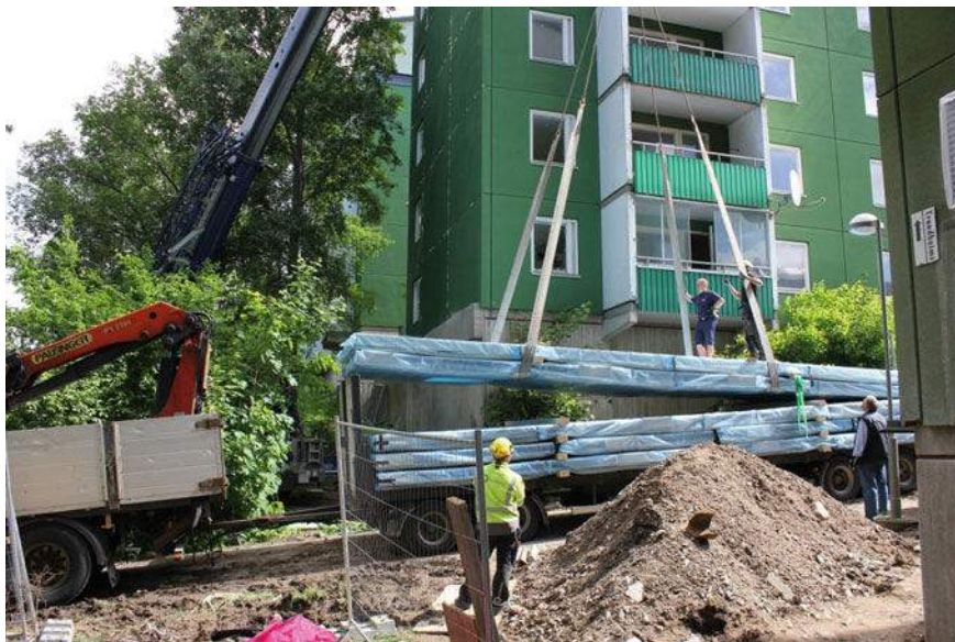
Fig. 4 Prefabricated elements arriving at the building site
