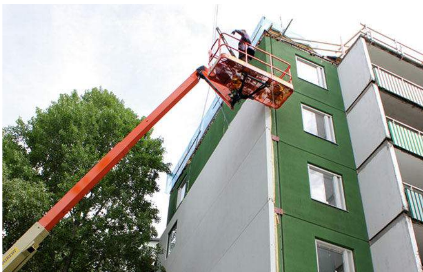
Fig. 5 Mounting of prefabricated elements was done with crane and sky lift
