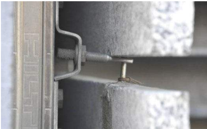
Fig. 3 Photograph of a stone panel with air chamber
