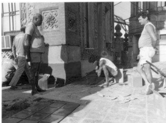
Fig. 11 Workers laying down the ceramic tiles on the fifth-floor terrace (1988)
