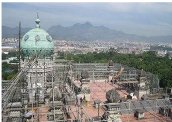
Fig. 24 Scaffolds on the seventh-floor terrace (May 2014)
