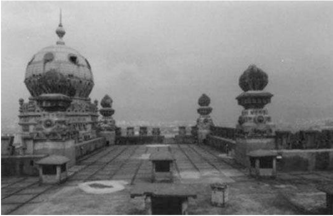
Fig. 7 View from the seventh-floor terrace, with the old cement tiles (1989)
