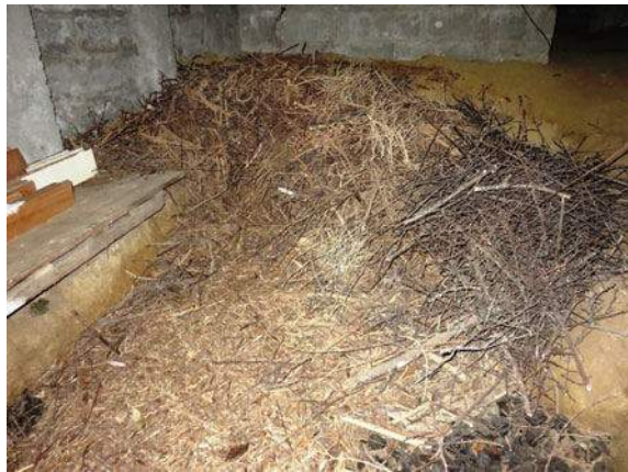
Fig. 4 Debris resulting from a nearby stream flooding
