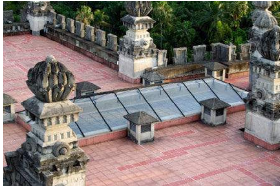
Fig. 15 View of the shelter dome on the seventh floor (Dec 2009)
