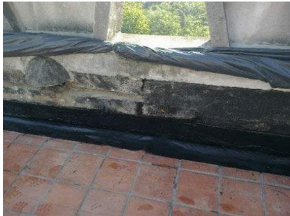
Fig. 25 Treating the edges of the butyl rubber blanket (Jun 2014)
