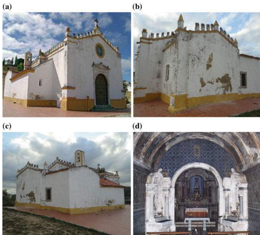
Fig. 3 Our Lady of Conception Church: a northwest view; b southeast view; c northeast view; d interior view
