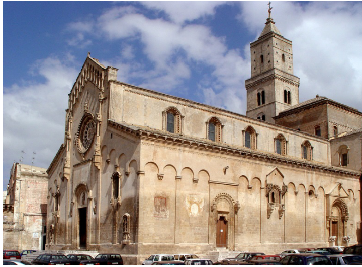
Fig. 1. The Matera Cathedral (exterior)
