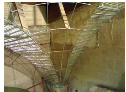
Fig. 17 and 18: Construction phases of the decorated star vault with pernevometal
