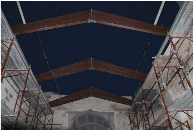
Fig. 15 and 16: Constructive steps: new covering
