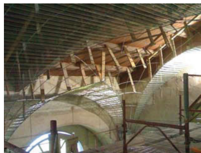
Fig. 17 and 18: Construction phases of the decorated star vault with pernevometal
