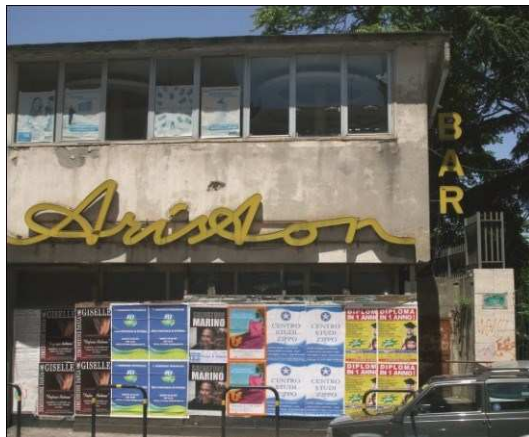
Figure 3. The Main Facade.
