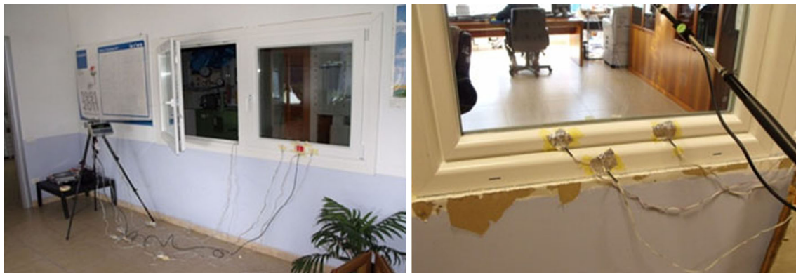
Fig. 6 Installation of the system and sensors for testing on-site
