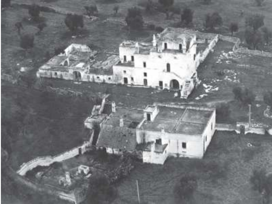
Figure 3. Masseria San Domenico before refurbishment (Source: Mongiello, 1996).
