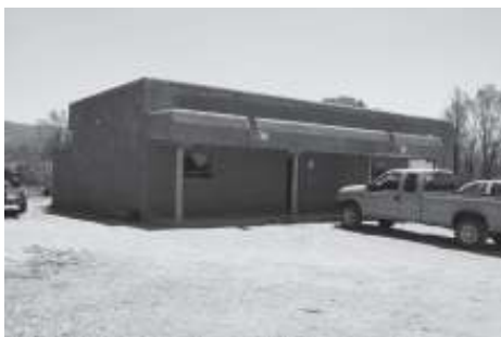
Figure 1. Taos Pueblo Preservation Program training center.
