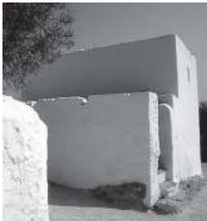
Figure 1. Typical house in Ibiza.
