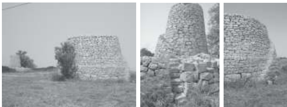
Figures 6, 7, 8. Ragusa, “Tre Bastoni” district. The “muragghi” with spiral staircases tower in the plot.
