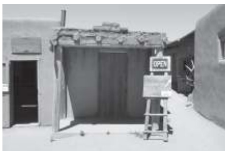
Figure 3. The adaptability of the adobe houses in Taos Pueblo to new uses, such as gift shops, indicates one of the aspects of the property's inherent sustainability qualities.
