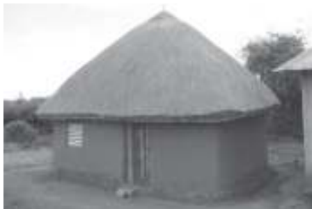
Figure 4. Illustrates a finished traditional house (Ojoo, 2009). The roof is made of thick layers of fine grass. The mud-walls are continuously smeared with red mud and cow dung for aesthetic purposes and protection from pest. In the past doors were woven with reeds and tough animal hides. But currently Iron sheets are preferred, mainly, to ensure security. 3
