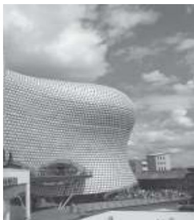
Figure 3. Department store Seldfridges.
