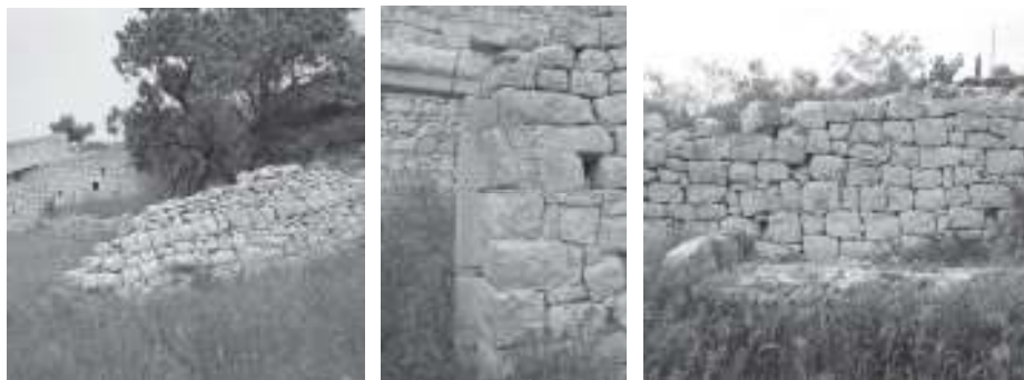
Figures 12, 13, 14. Details of the separating wall, the entrance door and the manger.
