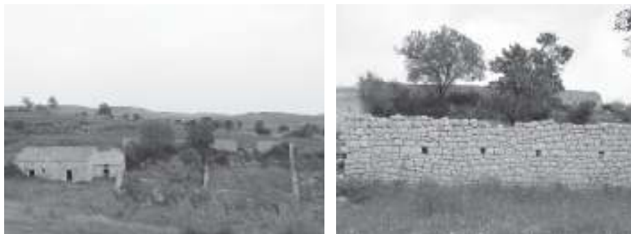
Figures 10, 11. Ragusa, “S. Margherita” district, Rural complex and “mannira” with double corral.
