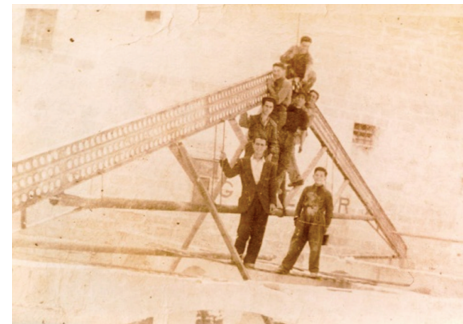
FIGURE 5: Historical image of iron trusses.
