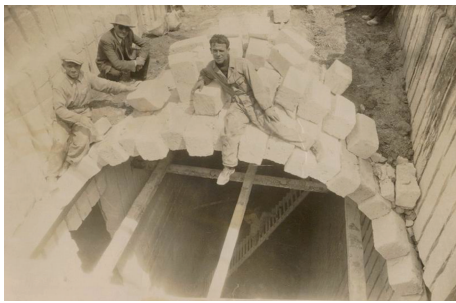
FIGURE 4: Historical image of vault construction.
