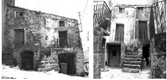
Figg. 5, 6 Entrance systems with external staircase
