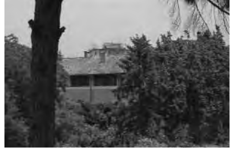
Fig. 3 An example of typical roof in the Vesuvian Area (Image: Archivio Mollo/DIC)
