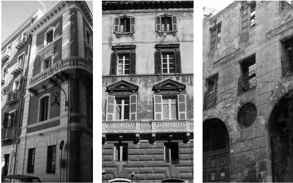
Final table for the comparison of the case studies. On the left: Palazzo Carboni-Boi Centre: Palazzo Barrago, On the right: Palazzo Aymerich
