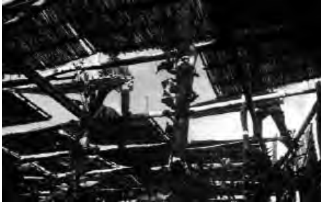
Working laying of pagliarelle
