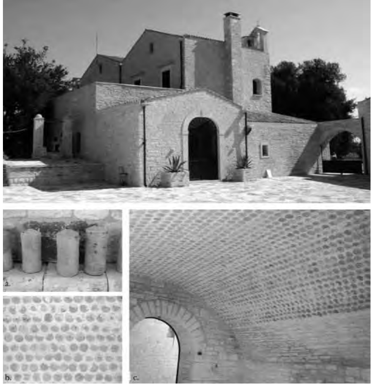
Fig. 1 - Masseria Spada, Corato (Bari). Typical vault in stone and "bubbole"
