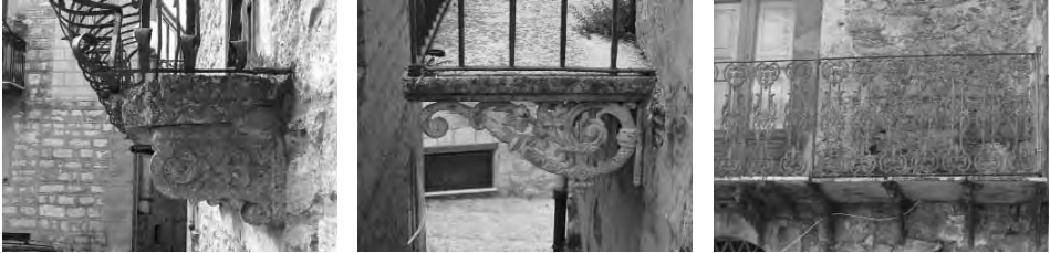
Figg. 7, 8, 9 - Stone and cast-iron brackets and balcony railing
