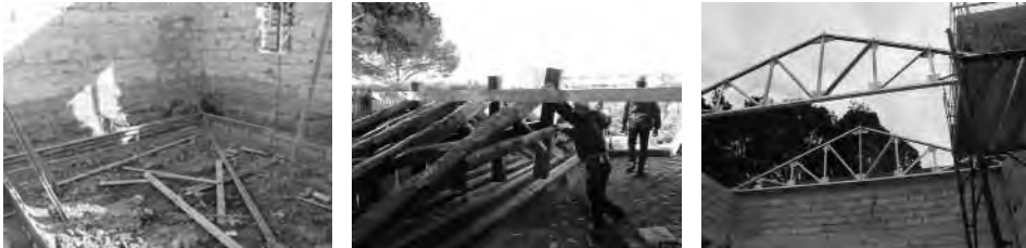
Fig. 6,7,8 - Some images of the building site
