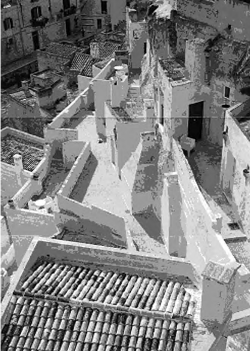
Fig.2 - Locanda of S.Martino (after the intervention)
