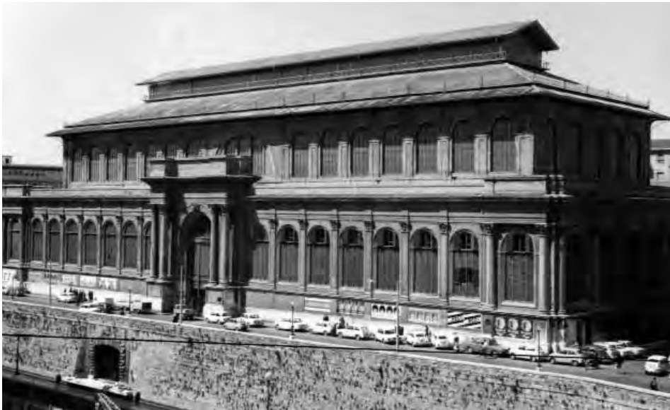
Fig. 2 (top) - View of the Market from the Royal Ditch
