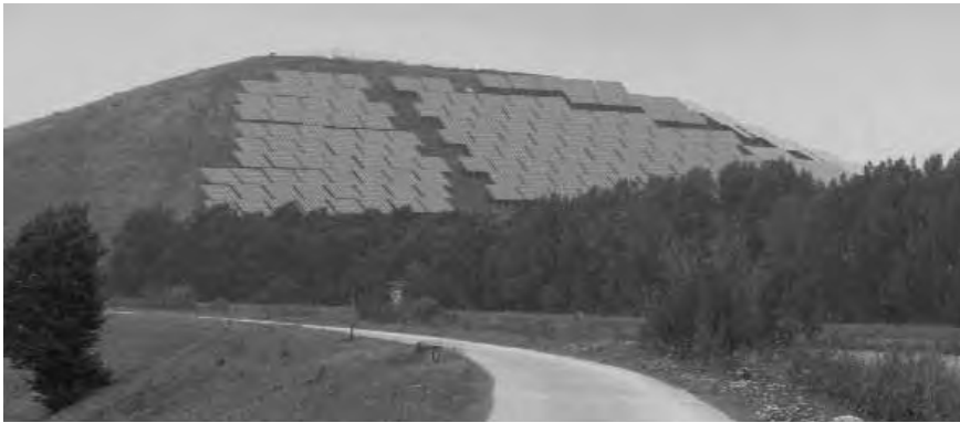
Fig. 2 - The photovoltaic system on the southern slope of the hill Atzenhof-Muellberg at Furth, Bavaria
