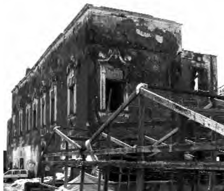
Fig.3 - North-West façade view
