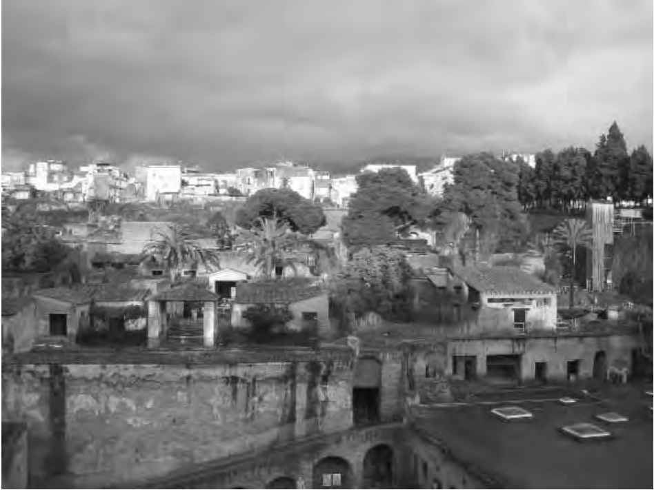
Fig. 7 - Roofs currently in use at Herculaneum. (Image: Studio Pesaresi/HCP)
