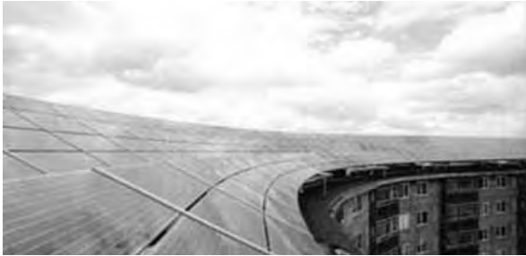
Fig. 4 - Plant-integrated photovoltaic roof of a residential complex in Denmark
