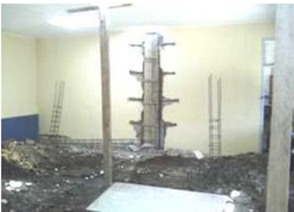
Fig. 6 Retrofit work of School Building I (ITB ).
