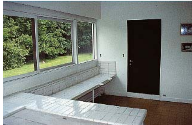
Fig. 3 In Villa Savoye of 1928, the kitchen is designed in line with the contemporary ideals of clinical hygiene. Everything is white and the tiles on the kitchen table are easy to clean.
