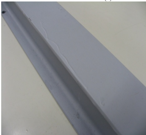
(b) Main girder without damage
