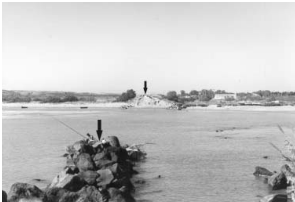
Photo 7 - Panoramic view of the Simeto River delta forming a mouth gulf. The black arrows indicate the artificial fluvial embankment, built with aim to constrain the seasonally flooding of the river, and partially eroded during last 10 years by the waves powerful action. Note the black basaltic blocks constituting them.
