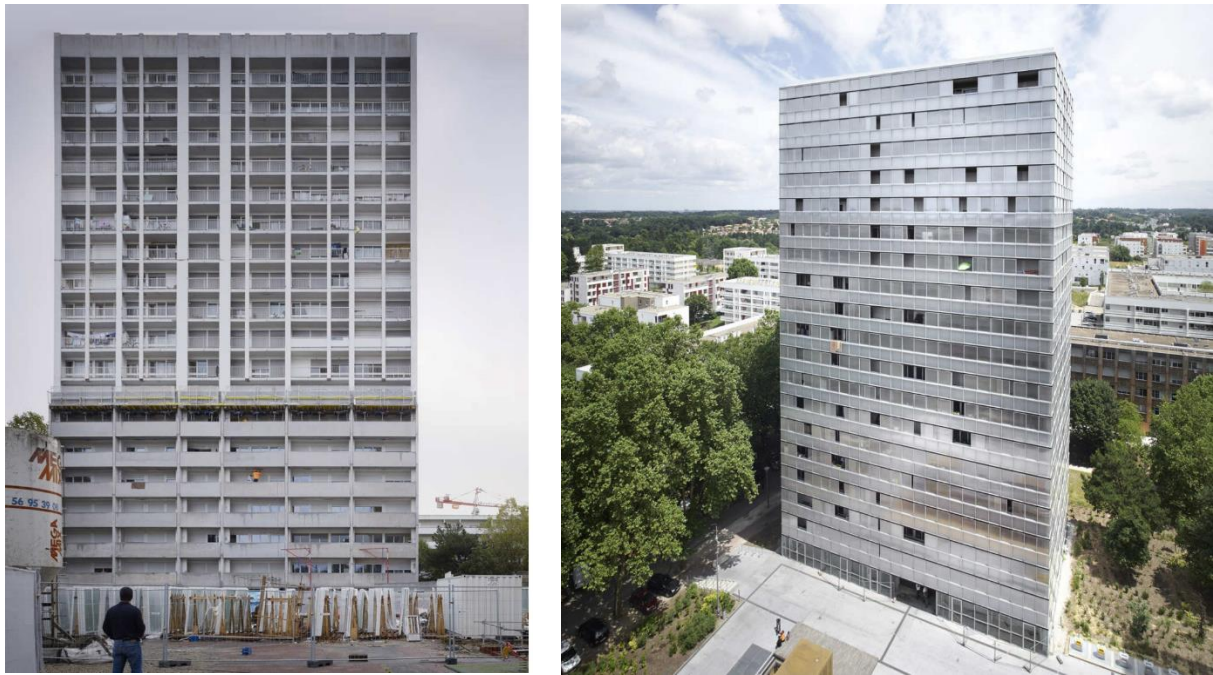
Fig. 2: Building before and after the façade renewal; (credit: LAN Architecture, www.lan-paris.com ).
