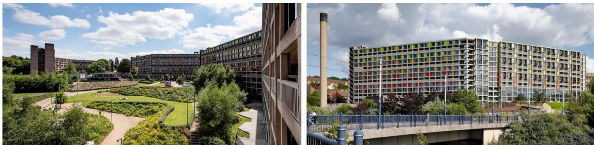
Fig. 5: Green space and new façade of Park Hill; Hawkins/Brown Architecture and Studio Egret West; (credit: Hawkins Brown Architecture, www.hawkinsbrown.com ).
