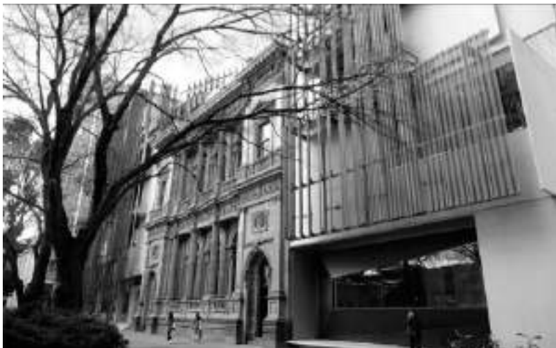
Figure 2. Image of heritage-listed Joseph Reed façade, originally fronting the Bank of New South Wales, at Melbourne School of Design. [Source: Google maps by Elliot Bledsoe, 2018].
