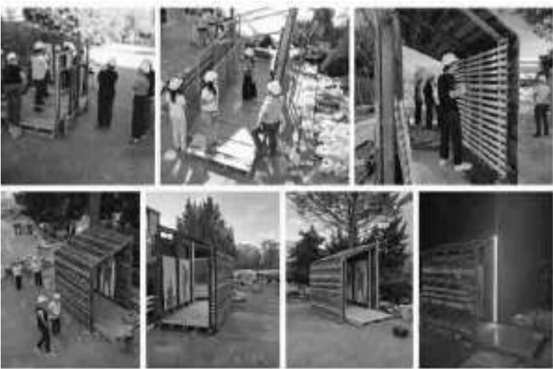
Figure 5. Assembly phases of the module during the workshop and construction site photography [Source: see Note 1].
