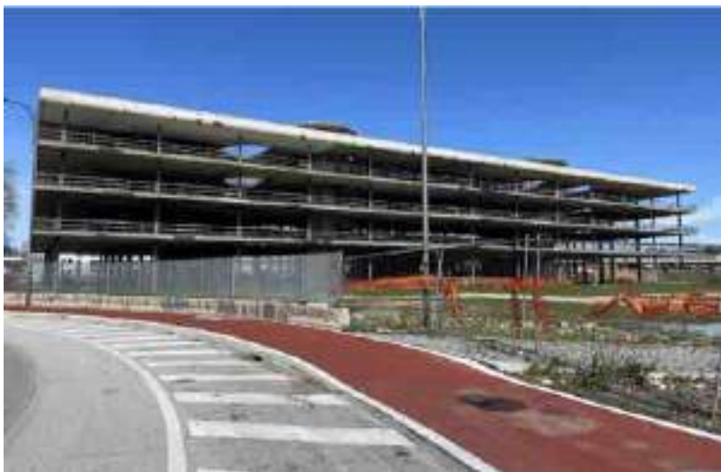
Figure 2. The unfinished reinforced concrete structure known as “La City”, Pescara located near the airport and the Cammino d’Abruzzo route. [Source: authors]. 1
