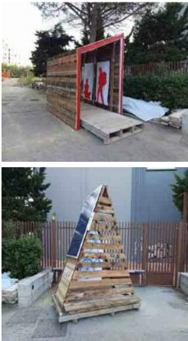
Figure 5. Two of the three modules realised during the HYLE summer school in Pescara, showing the use of recovered materials (wooden pallets, metal profiles) assembled with reversible mechanical connections. [Source: Note 1].
