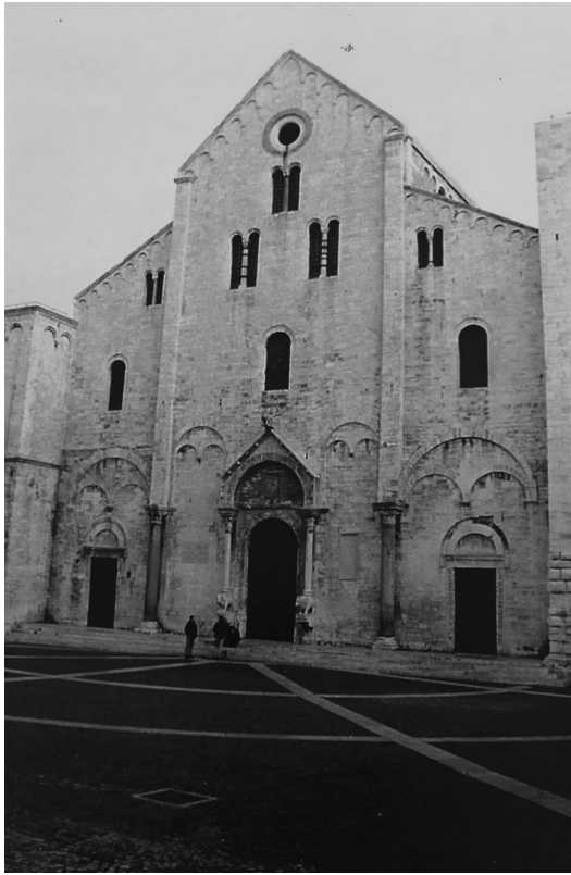
Fig. 3 1998, Basilica main elevation (west side) (A-SABAP-BA 1999)
