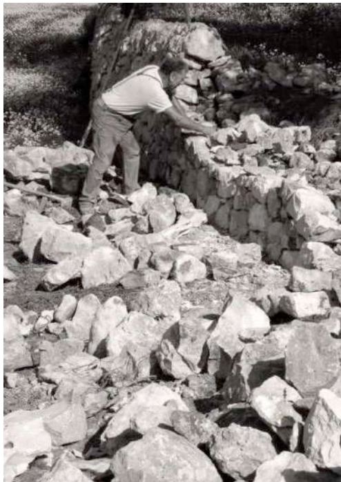
Fig.2,3,4 - Paolo Zaffarana, construction of a drywall. Source: Archive Giuseppe Bertucci.
