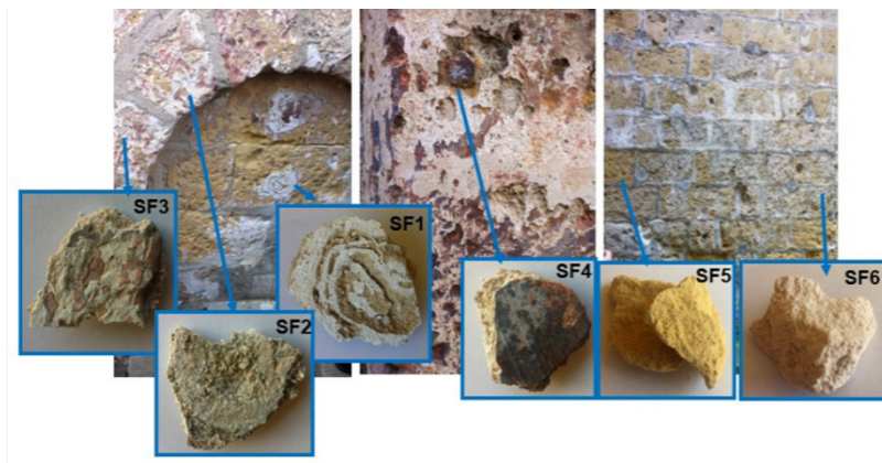
Figure 8. Sampling of the back façade of San Francesco d'Assisi.
