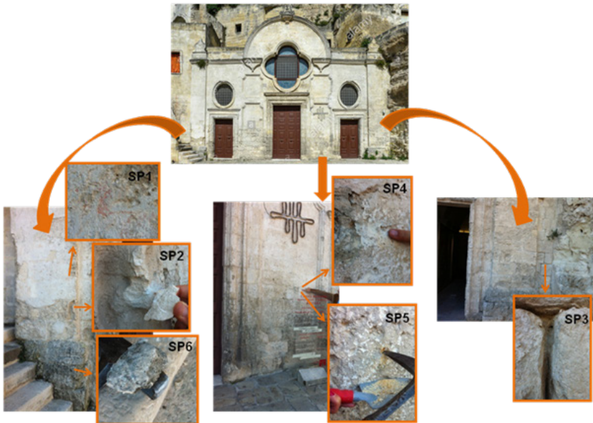
Figure 3. Sampling of the façade of San Pietro Barisano.
