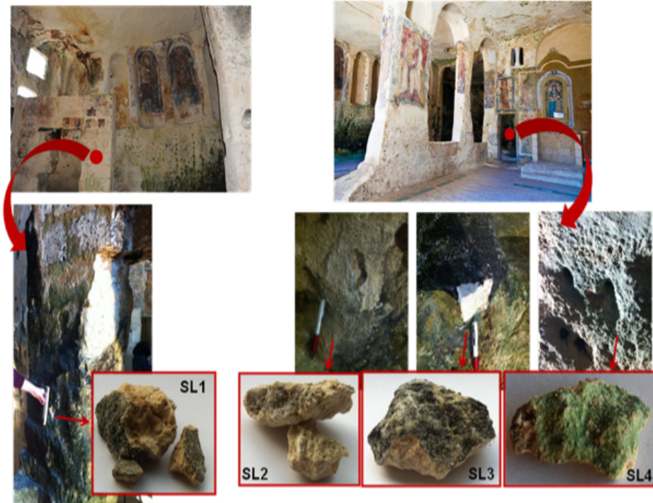
Figure 10. Sampling in the interior rock faces of the church of Santa Lucia alle Malve.
