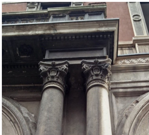
Figure 1. Example of black crust formation.
