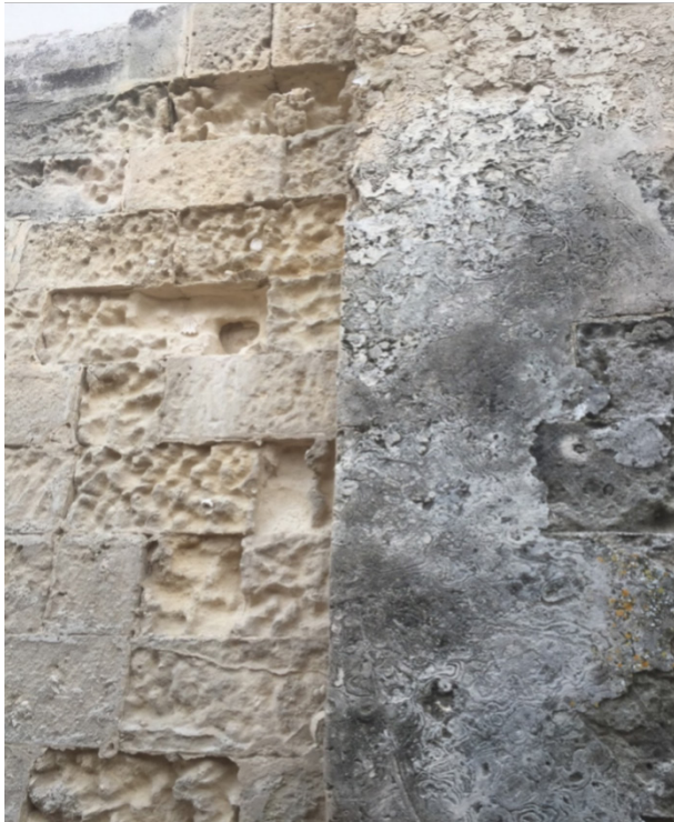
Figure 2. Detail of a masonry with varying degrees of alveolization of contiguous ashlars.
