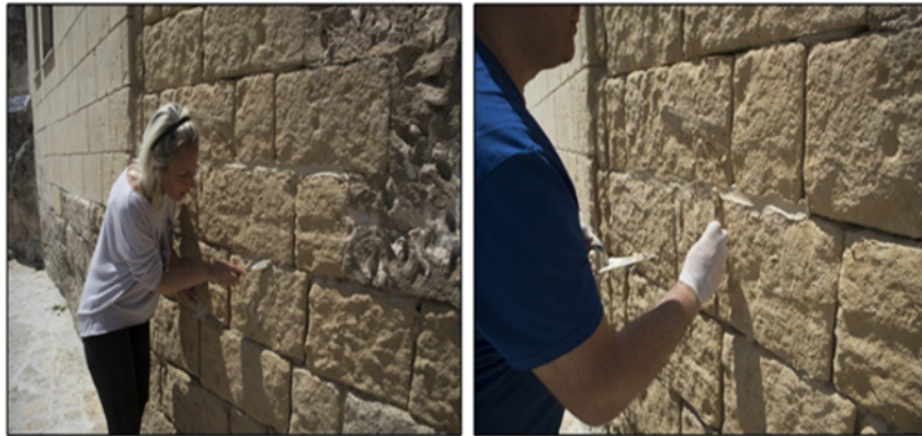
Figure 12. Remaking of the degraded joints in the sample area of the masonry of the bell tower of San Pietro Barisano with a pre-mixed commercial mortar based on lime and pozzolan.
