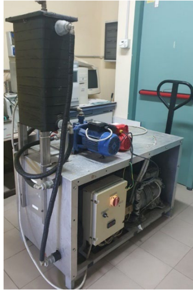
Figure 28 - Air-Cooled Chiller in the Laboratory Setup
