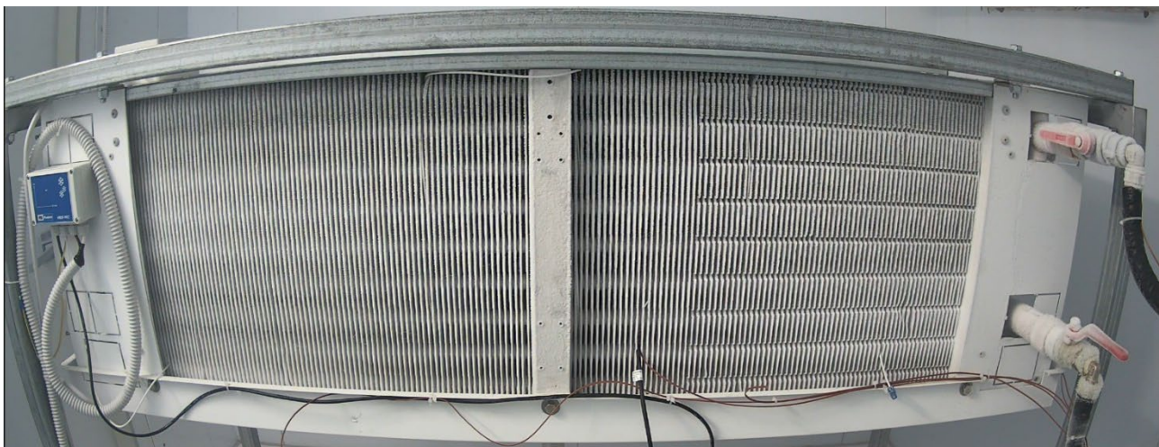
Figure 42 - Condition for defrost start (fan power consumption 250 W)
