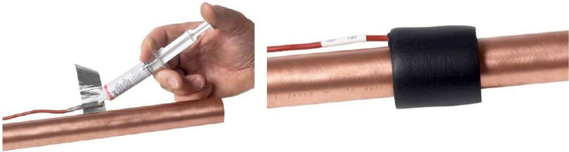
Figure 25 - Sensors installation using heat transfer paste, aluminum tape, and thermal insulation
