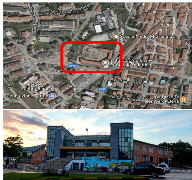
Figure 6 | Orthophoto of the intervention area and overall view of the M. Prezioso primary School.
