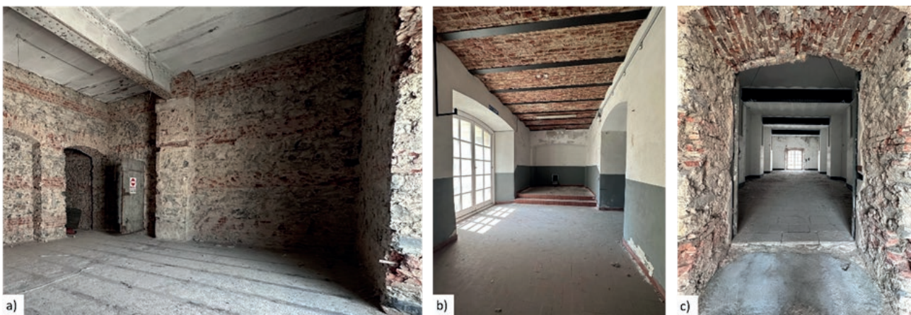
Figure 6. From left to right: a) masonry with courses of brick and Promontorio stone with the granite padstone where the floor beam ends; b) vaulted ceiling with metal joists; c) floor made with limestone elements. (Source: Authors).
